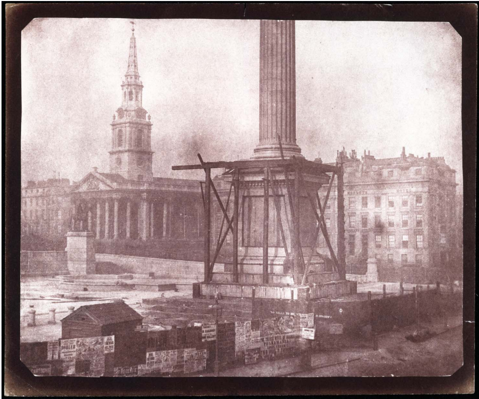
FIGURE 1 "Nelson's Column under Construction, Trafalgar Square, London", April 1844.
